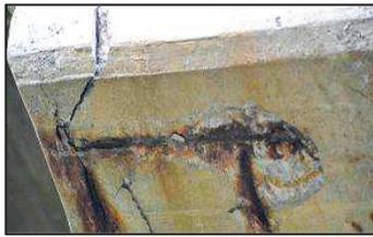
**Fig.1.** The effects of chloride on reinforced concrete
